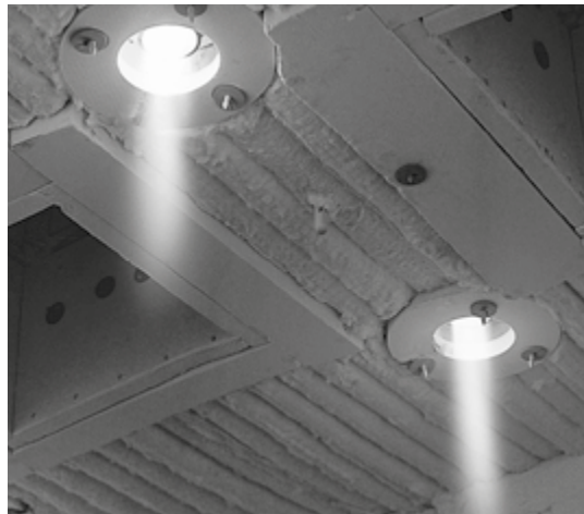
Overhead heating with burner BIC
