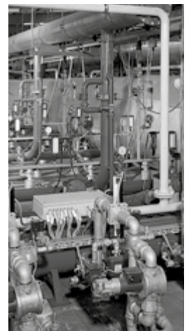
Tunnel kiln overhead heating
