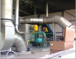
Exothermics was contacted by a major cheese manufacturer to provide an air heater that would deliver clean, heated process air for the operation of a new whey spray dryer. Exothermics' solution was a pair of Eclipse ER Indirect Air Heaters operating side-by-side. Not only do these air heaters produce clean hot air for this customer, free of combustion by-products and other contaminants, but they do so with impressive fuel efficiency.
