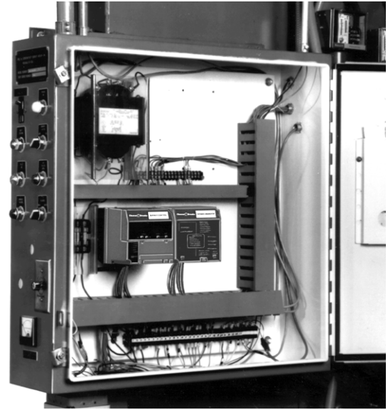
Fig. 5. Electrical panel installation.
